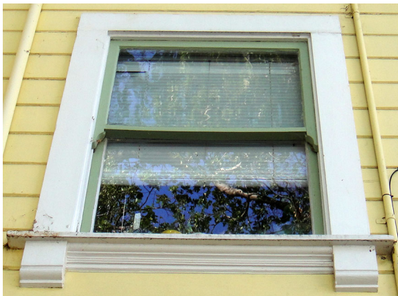
Figure 20. Mid-story window on east façade
