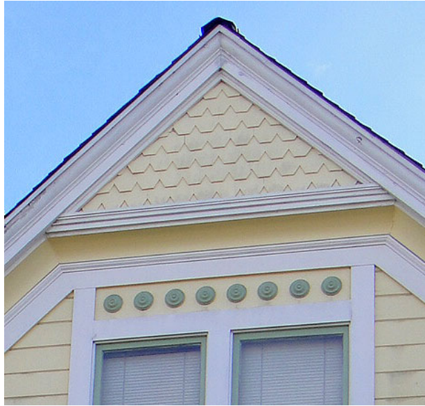
Figure 10. Front gable details
