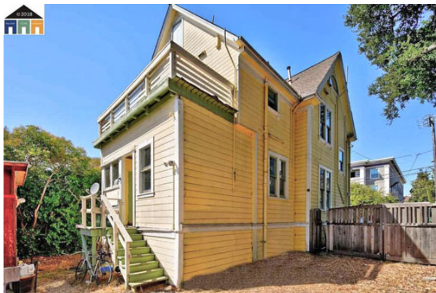
Figure 22. East façade & rear addition (realtor.com, 2018)
