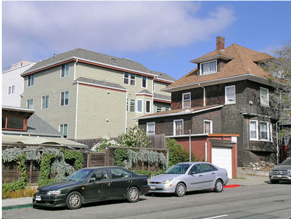
Figure 96. 2414 (left) & 2418 Dana Street, seen from Haste Street
