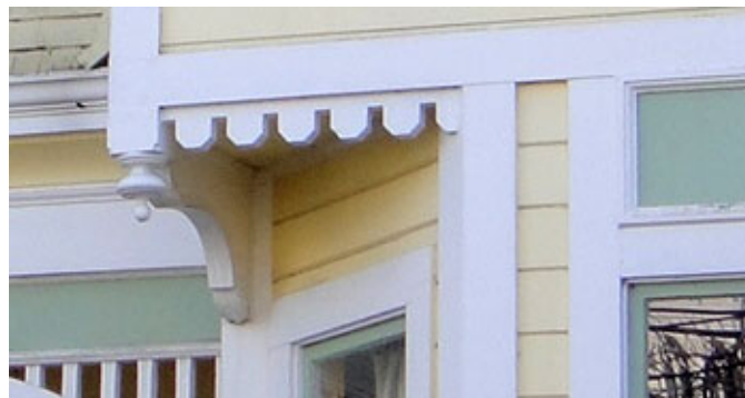
Figure 11. Scalloped edge & finial over bay window
