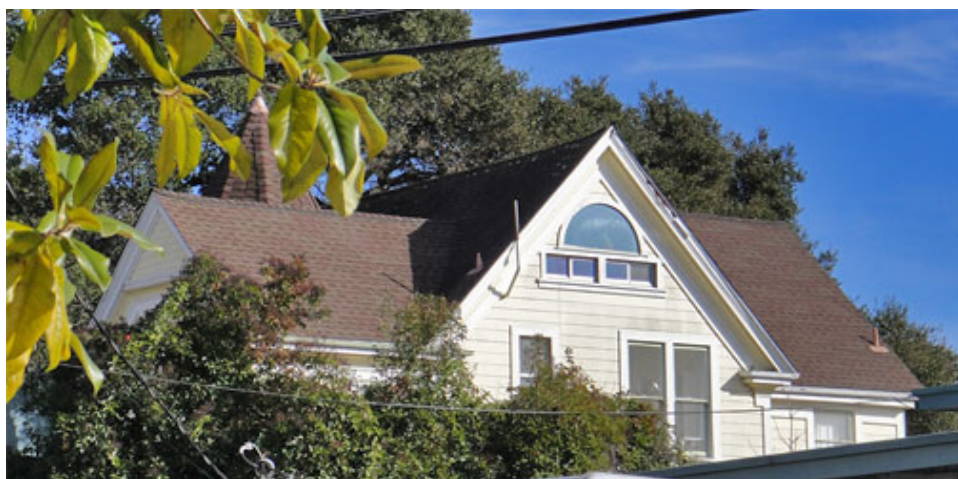
Figure 23. Upper west façade
