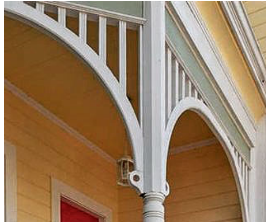
Figure 17. Porch arch detail (Realtor.com)
